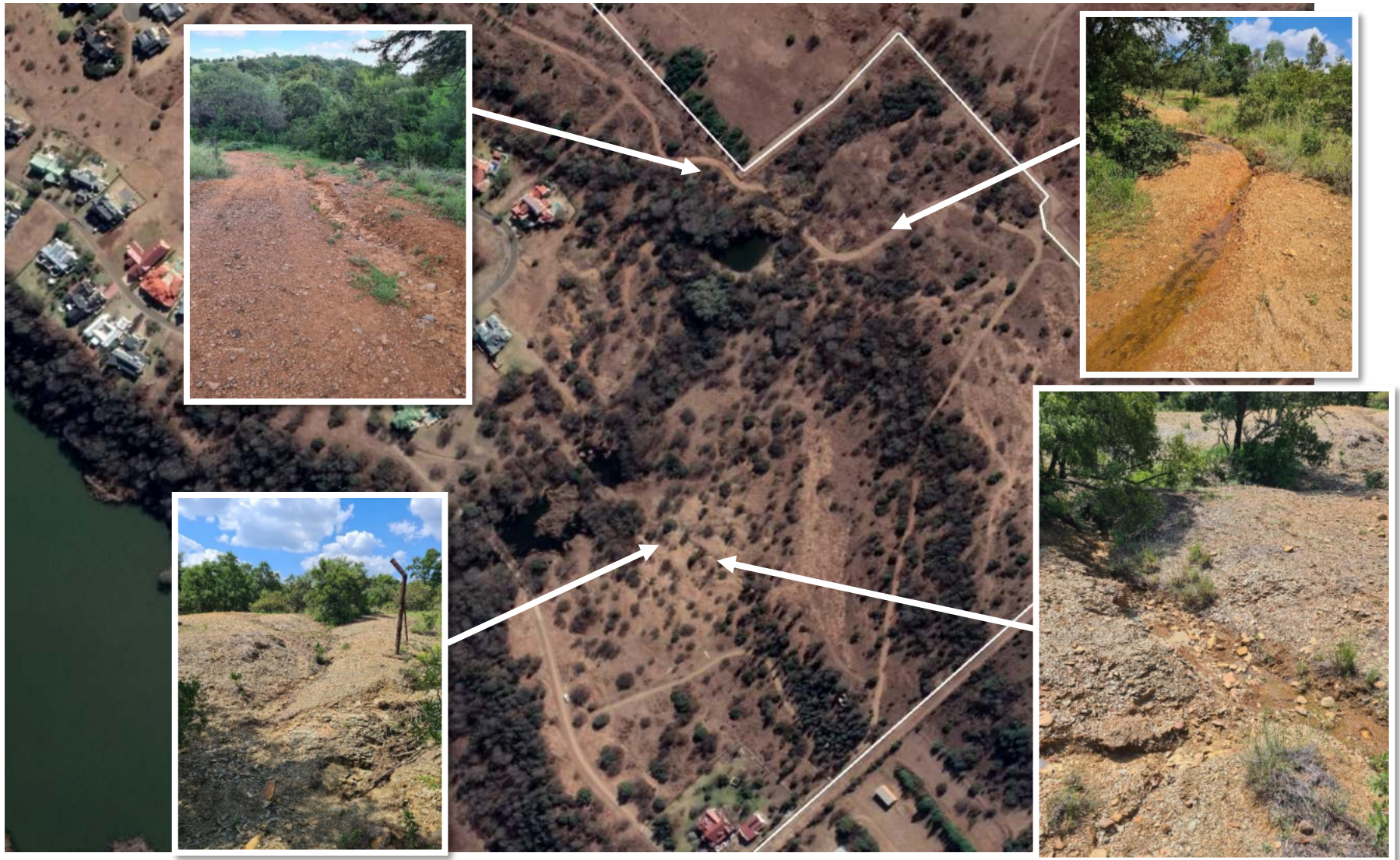
Figure 16: Areas where erosion is taking place on the estate
